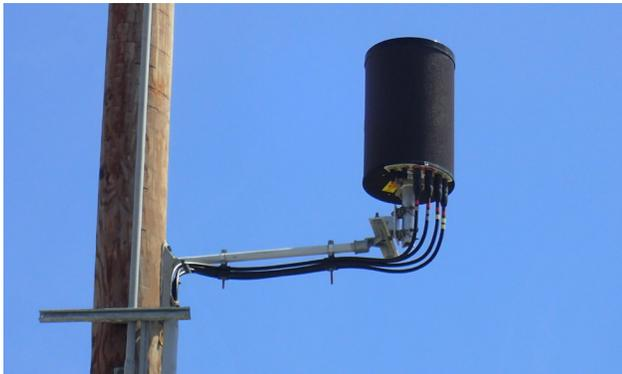
Small cell deployments to support 4G network densification in preparation for 5G are accelerating. Tens of thousands of small cell nodes are anticipated to be installed over the next several years. To accommodate municipal codes and technology changes, small cells can take on multiple form factors and architectures. Connecting the antenna and radio may require different sizes, types and lengths of coax and connectors depending on the site configuration and radio equipment manufacturer.
